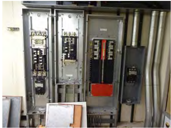
3 rd Floor Computer Lab – Electric Removed
