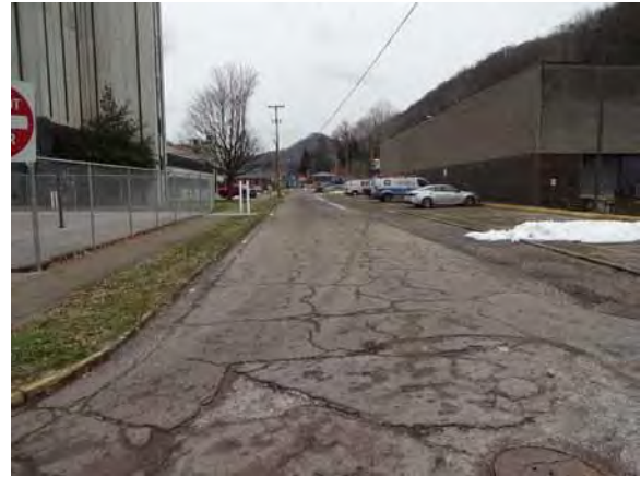
1 st Avenue Looking East
