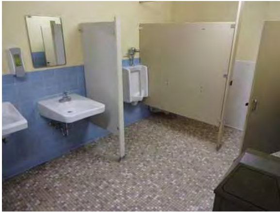
Mezzanine Men's Restroom
