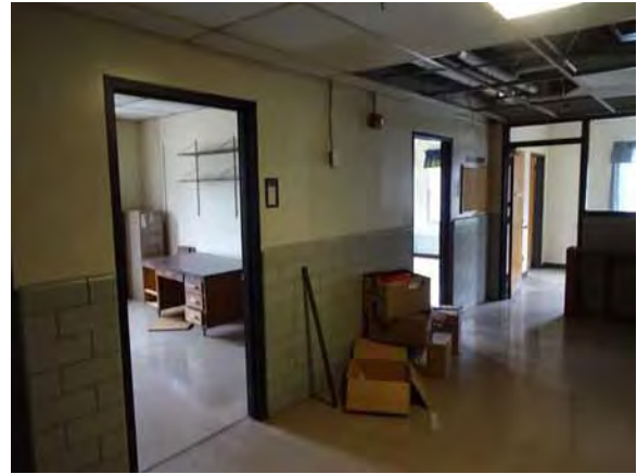
6 th Floor Hallway
