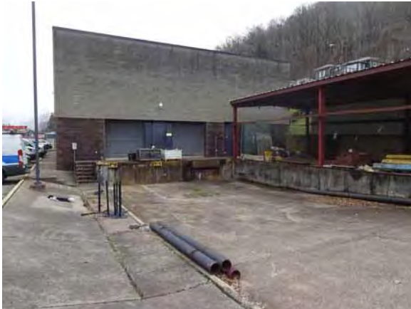
Truck Dock on West Side of Building
