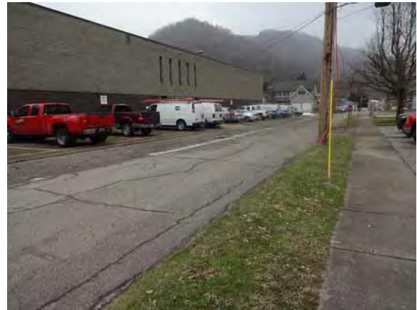
1 st Avenue Looking West
