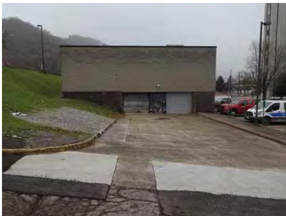
Garage Access on East End of Building
