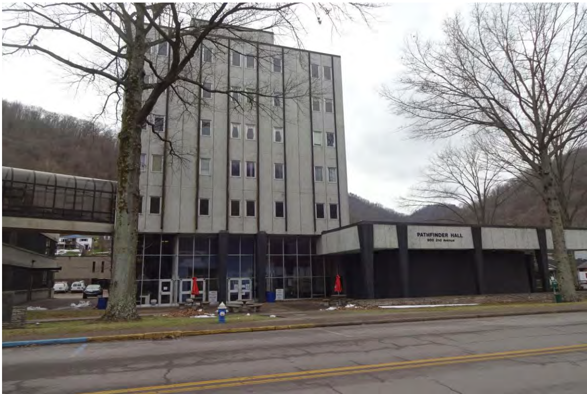
Pathfinder Hall Building
